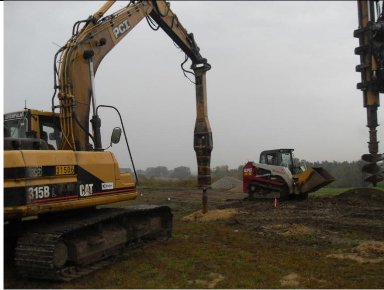
Figure 51. La Port City field conditions
