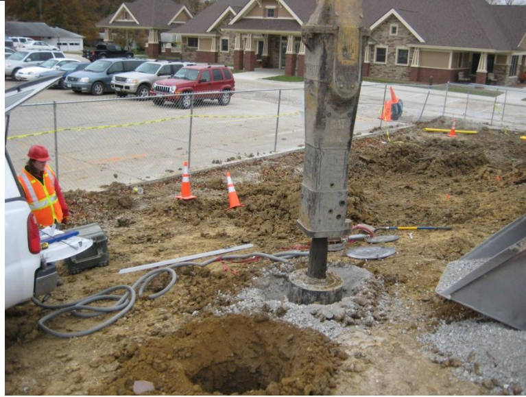
Figure 73. Oskaloosa field study conditions
