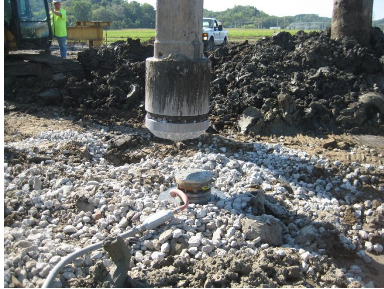
Figure 67. Council Bluffs field study conditions
